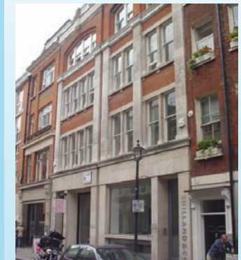
56a Poland Street, WC1 Various floors let to Reliance Media Group
