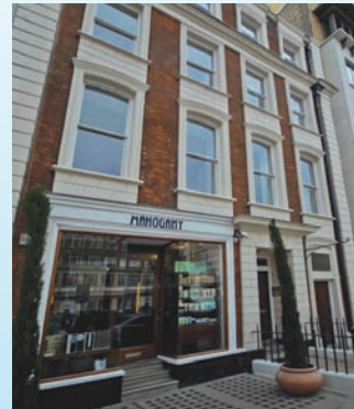
17 St George Street, W1 Entire upper part let to Faberge
