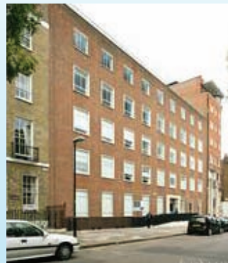
Bedford House 21A John St WC1 Part ground floor let to Steeles Law
