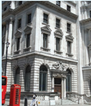
7 Waterloo Place, SW1 Lower Ground/Ground Floor let to Sofitel
